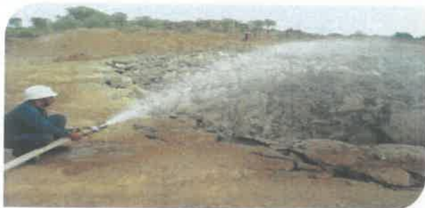
WATER SPRINKLING ON BLASTED MUCK
