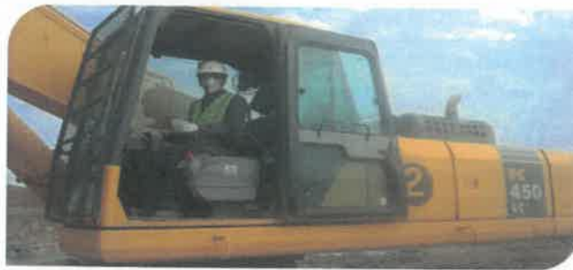
USE OF PPEs BY EXCAVATOR OPERATOR
