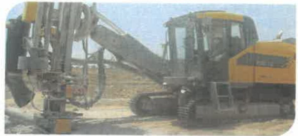
USE OF PPEs BY DRILL OPERATOR
