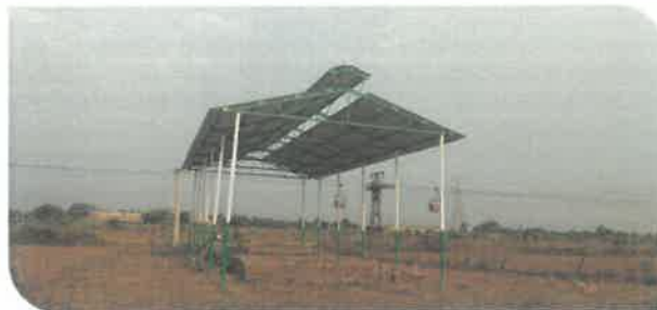
Road & shed Construction
